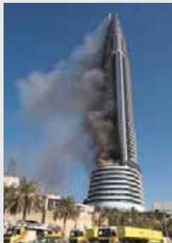
حريق THE ADDRESS HOTEL DOWNTOWN DUBAI
